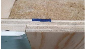
Q-panel with half-lap with insulation and adhesive tape.
